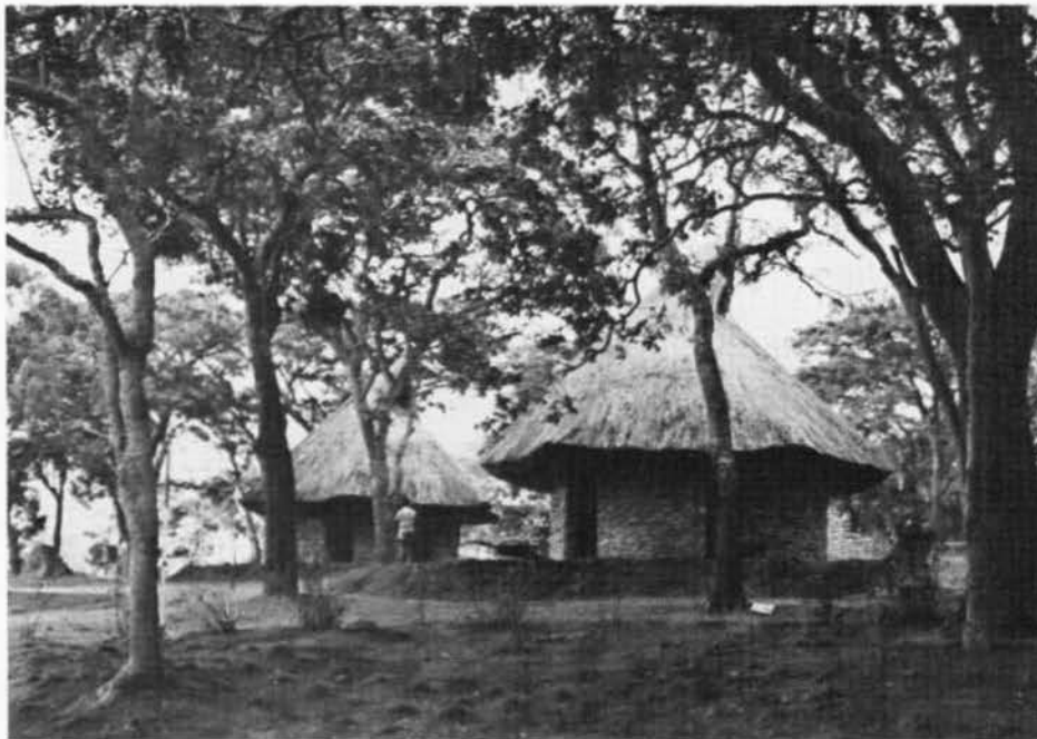
Housing for OTRAG employees.
