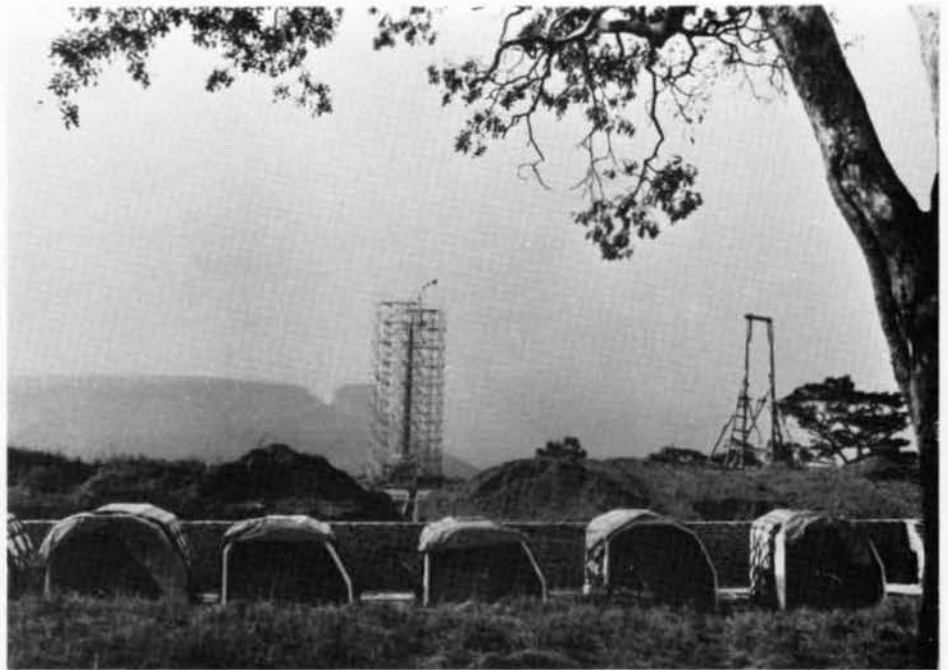
Propellant storage tanks in foreground contain nitric acid and kerosene. Center is the new gantry; to the right is a relic of OTRAG's earlier days.
