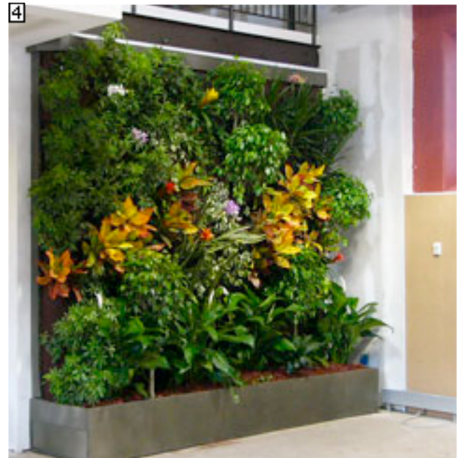
Living Wall installation, Baltimore, MD. This 110 sq ft (10 sq m) wall filters all the air for its 7,500 sf office building. Notice the ornamental character of some plants chosen
