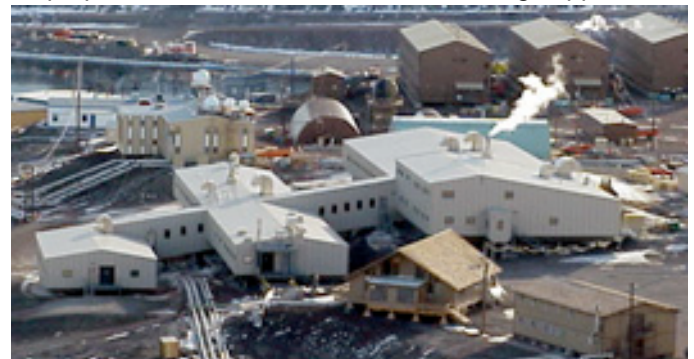
Albert P. Crary Science and Engineering Center, 1991
